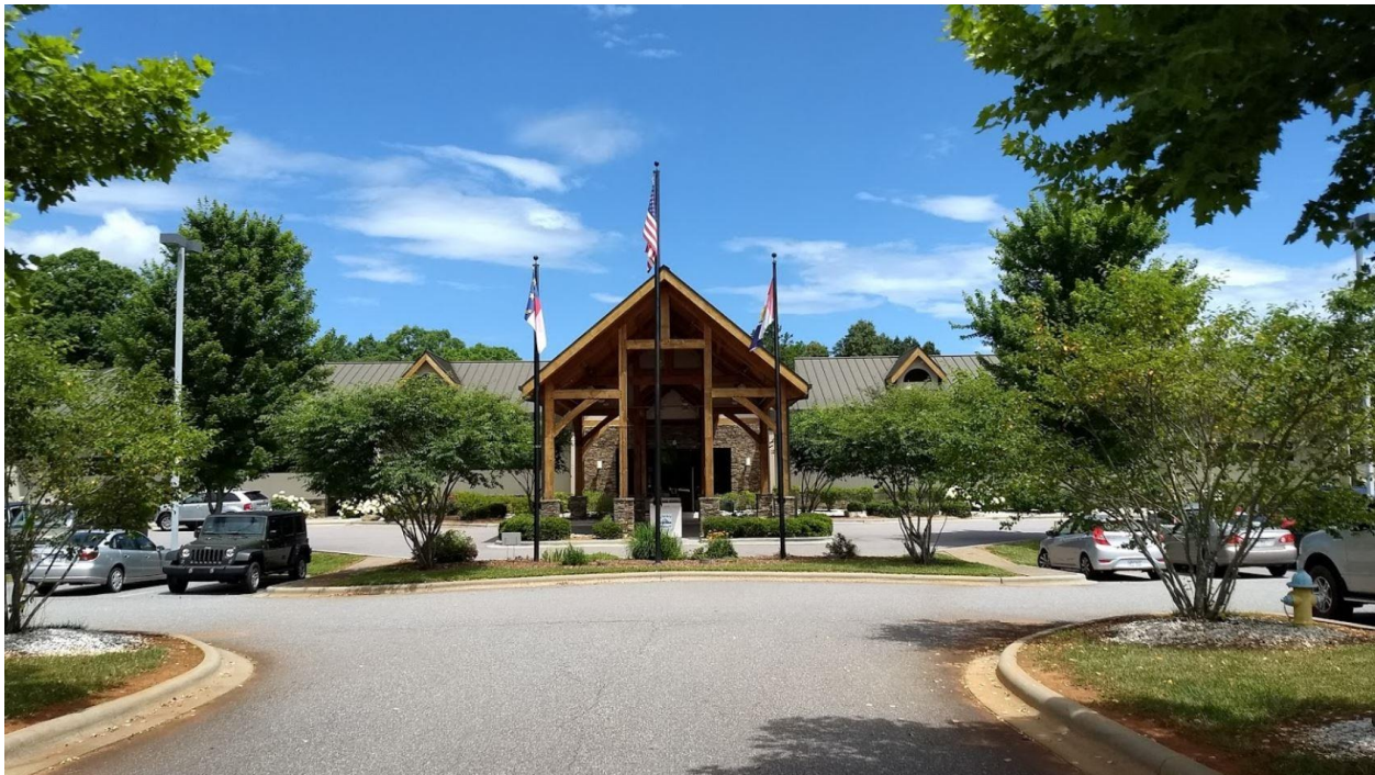
Fig. 1 – Overview of facility
