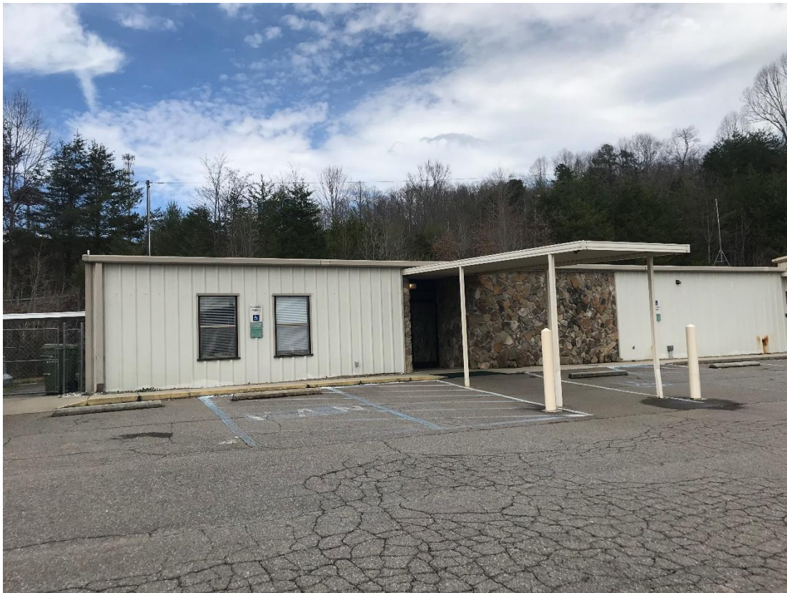
Fig. 1 – Overview of facility
