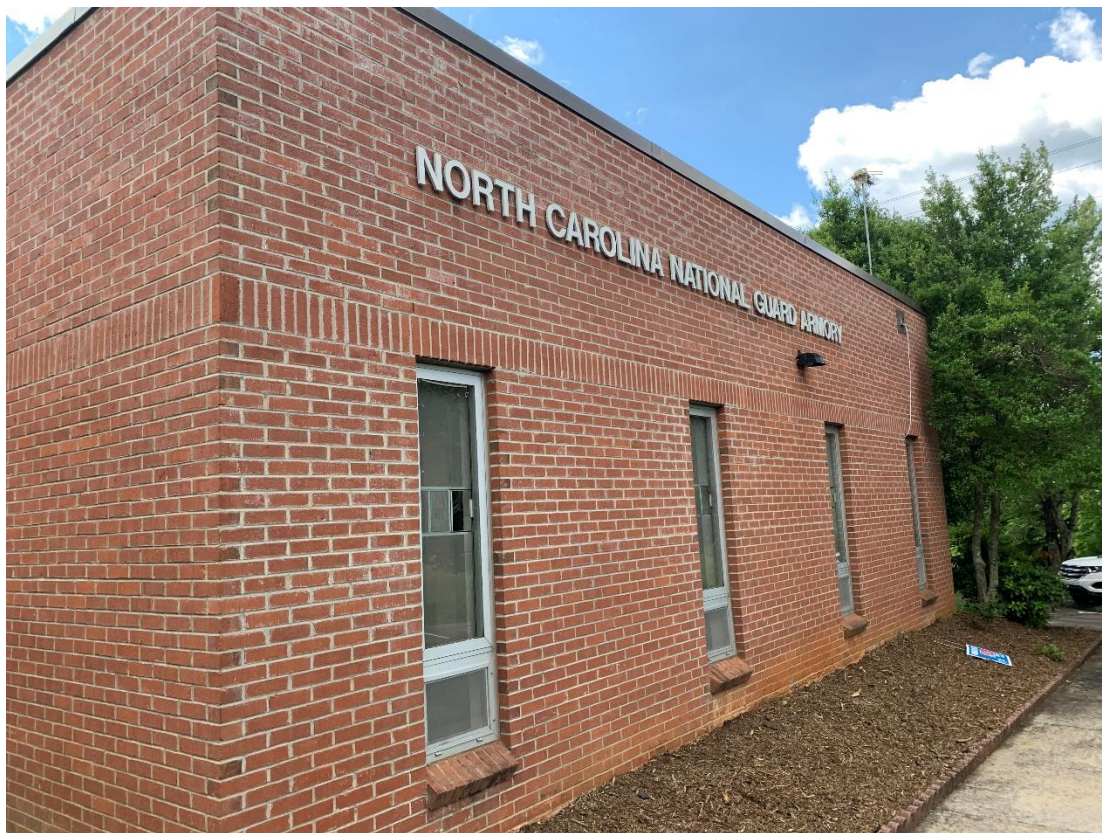
Fig. 1 – Overview of facility
