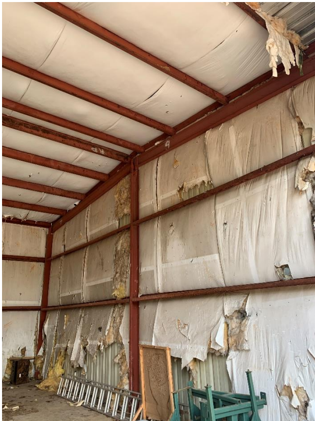
Fig. 2 – Deterioration in Armory Garage
