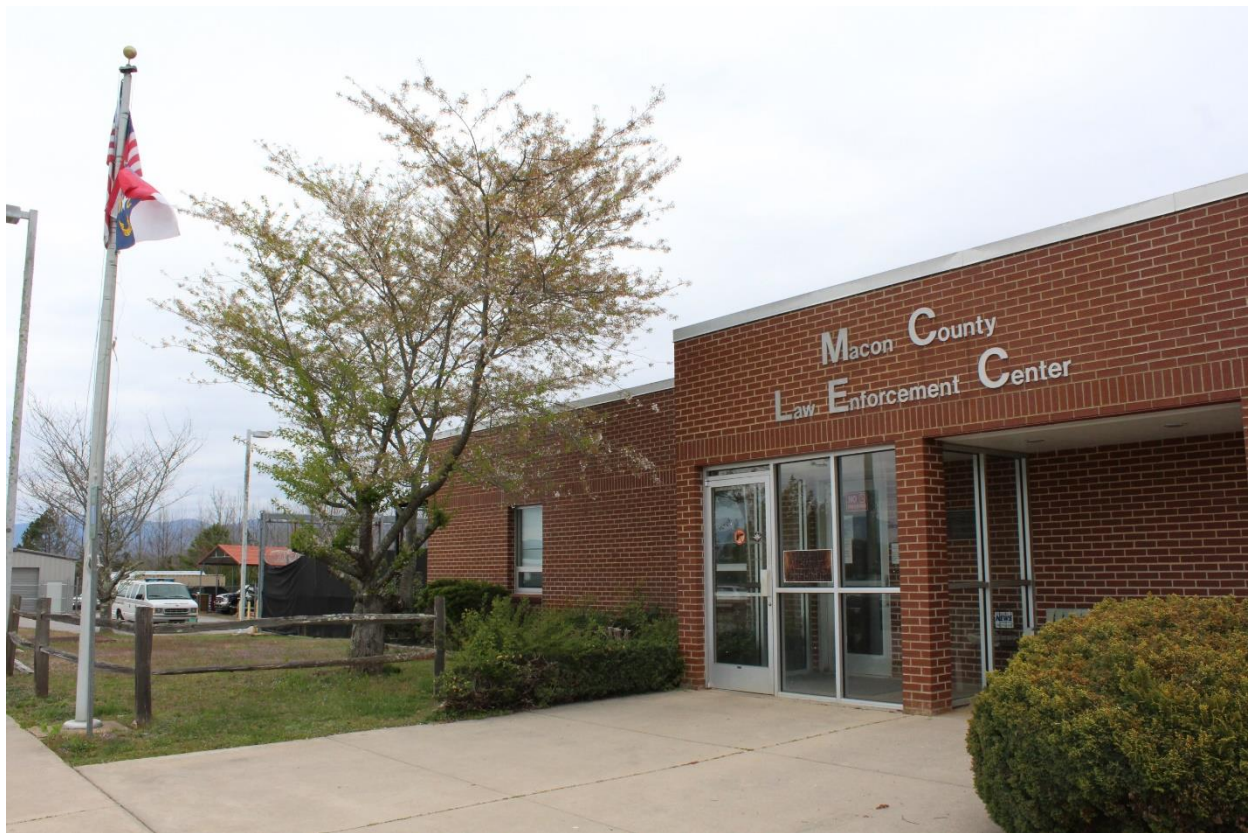
Fig. 1 – Overview of facility
