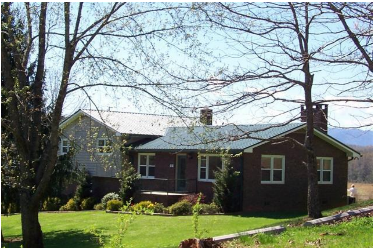
Fig. 1 – Overview of facility
