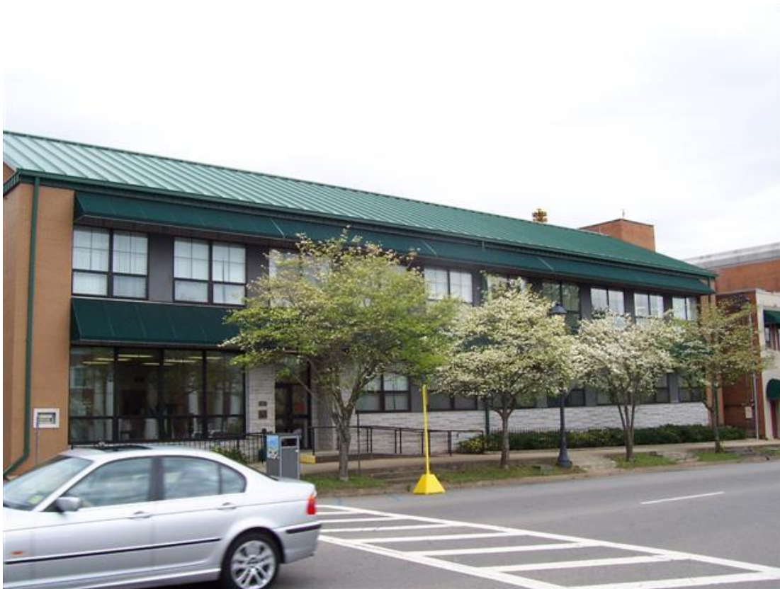
Fig. 1 – Overview of facility
