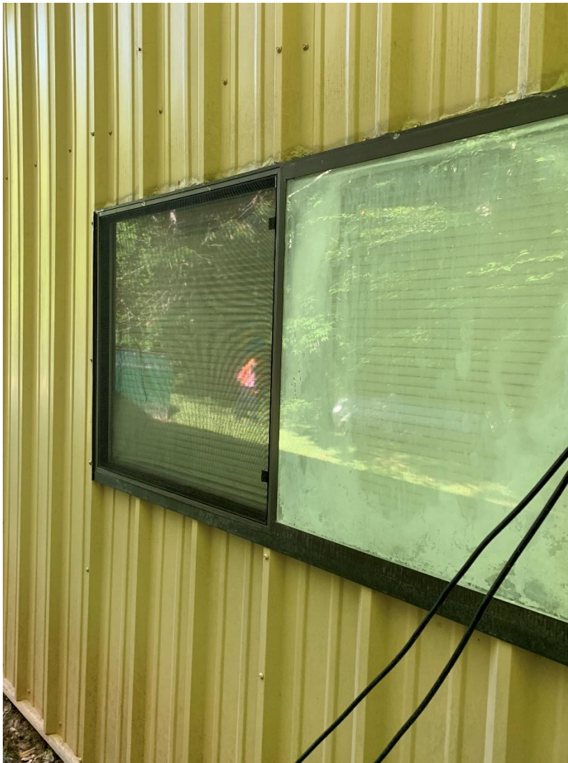
Fig. 2 – Window condensation
