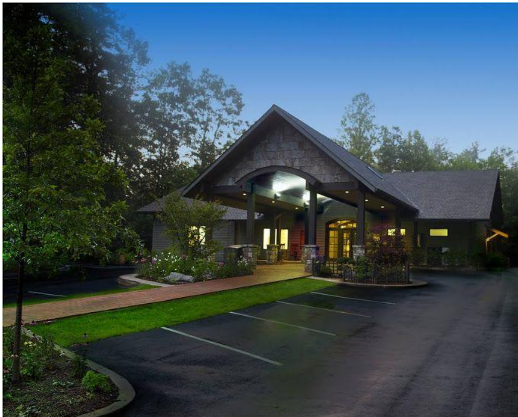
Fig. 1 – Overview of facility
