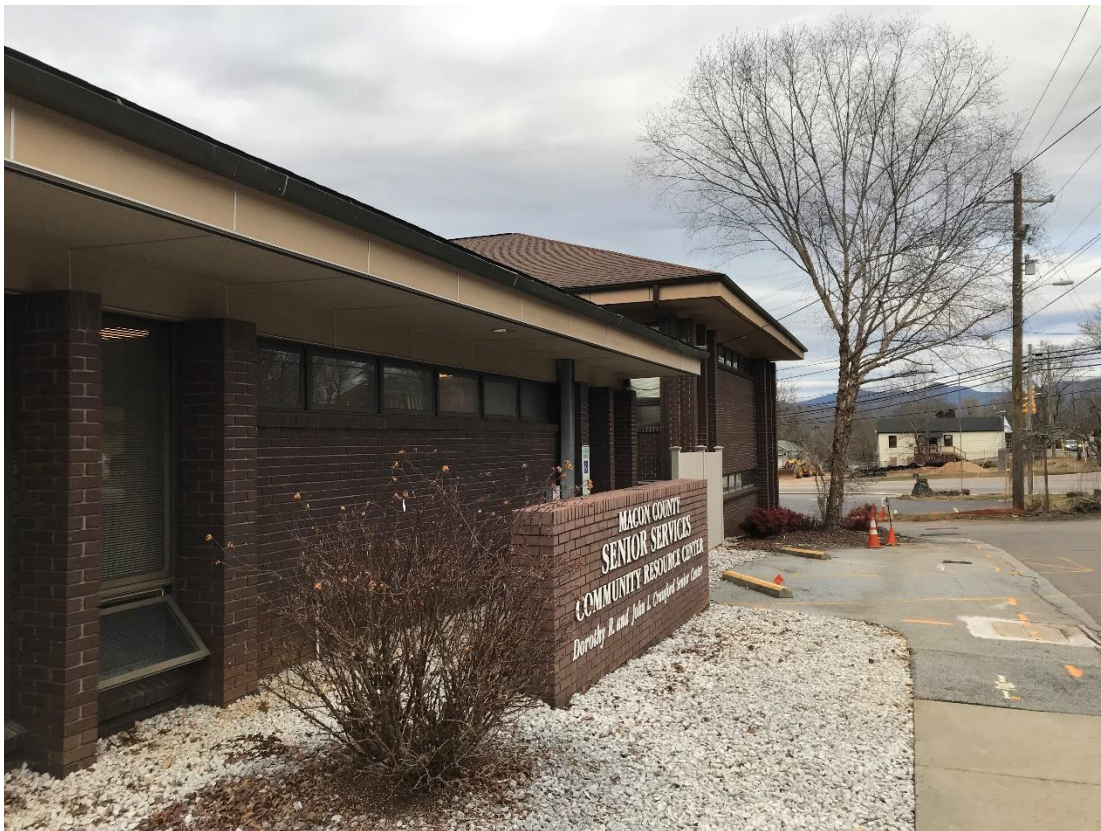
Fig. 1 – Overview of facility
