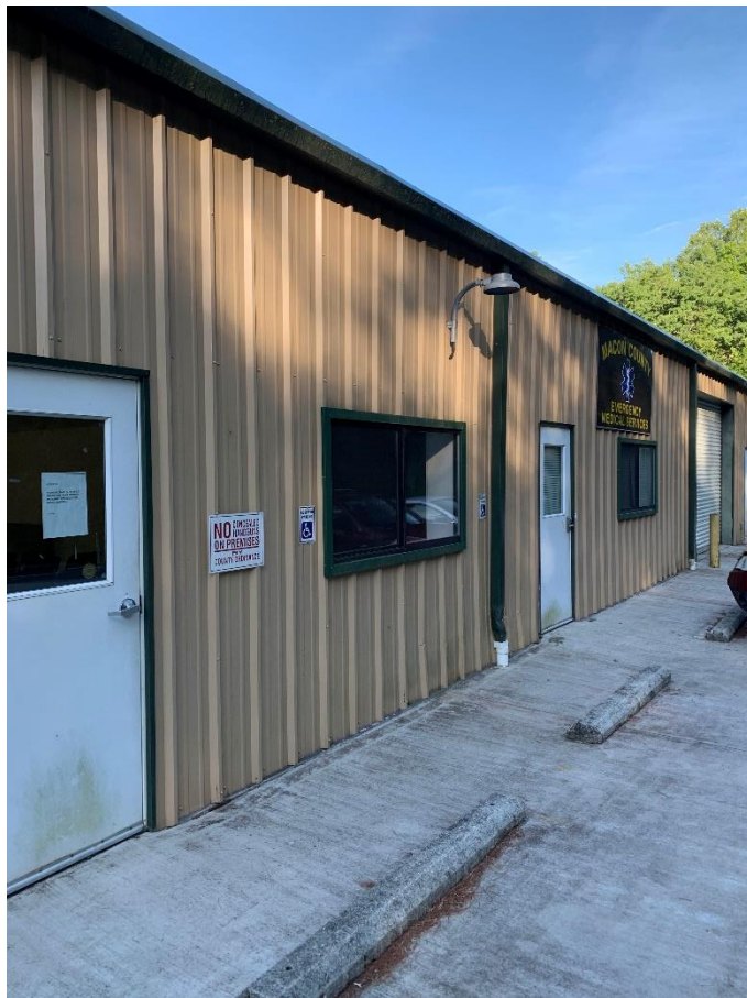
Fig. 1 – Overview of facility
