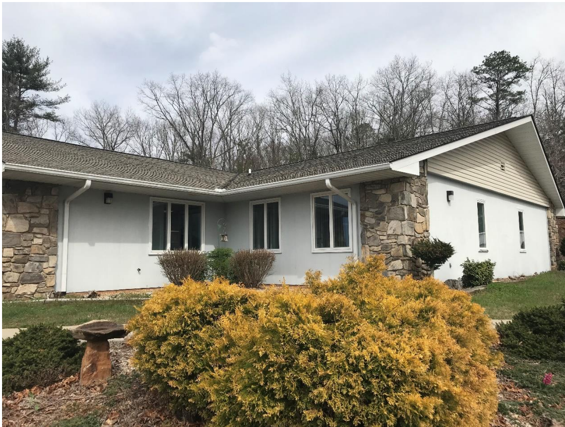
Fig. 1 – Overview of facility
