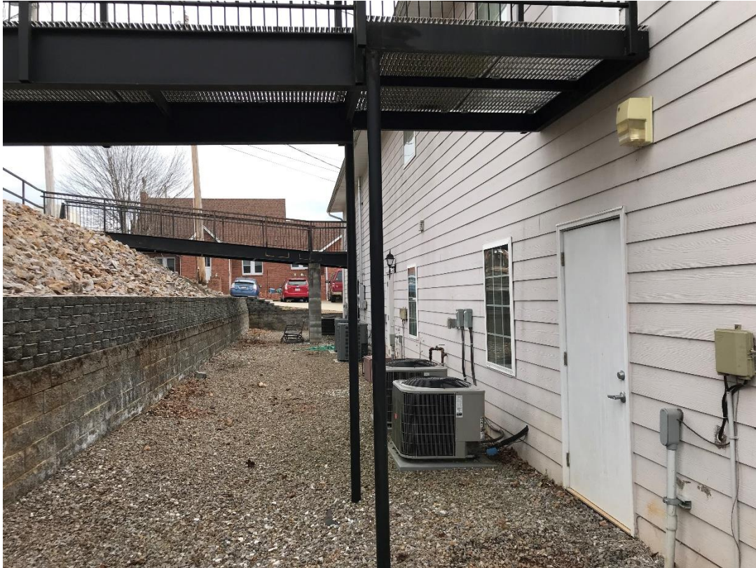
Fig. 2 – Overview of facility
