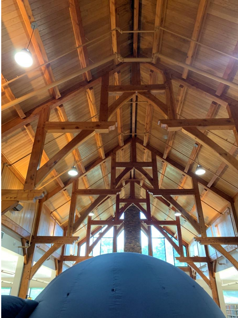
Fig. 2 – Timber frame interior
