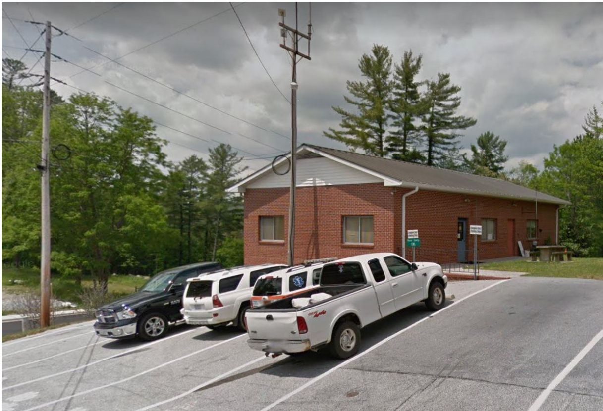
Fig. 1 – Overview of facility
