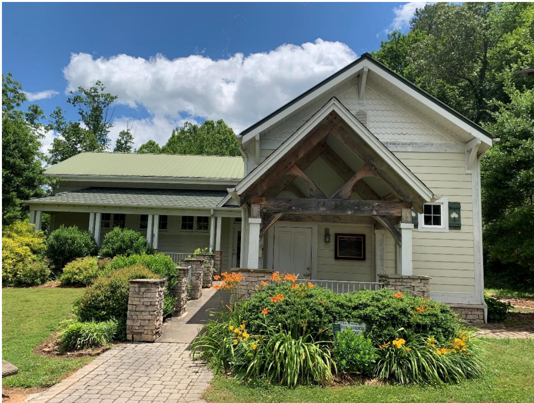
Fig. 1 – Overview of facility
