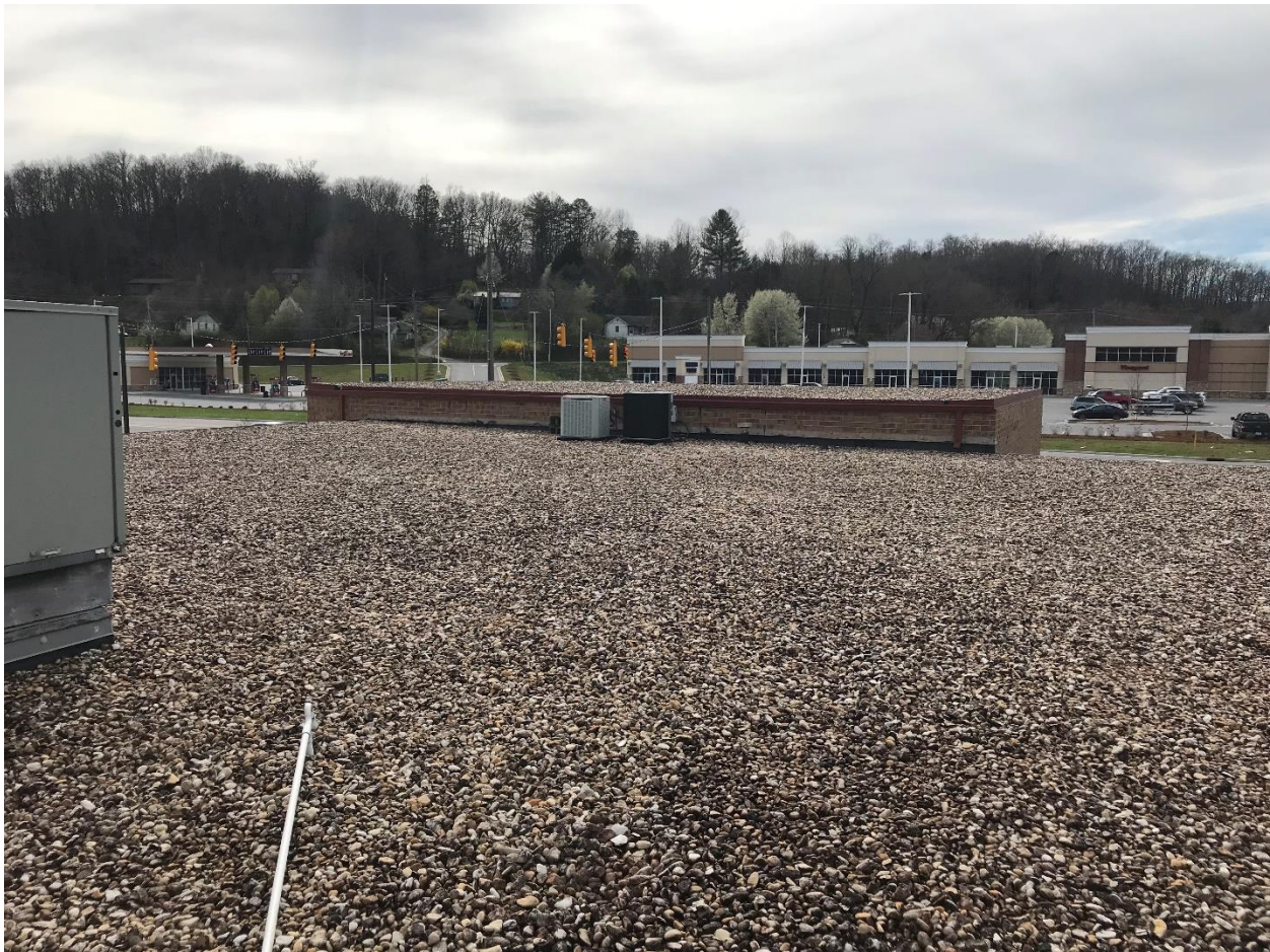
Fig. 2 – Ballast Roof System
