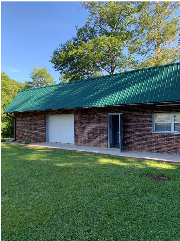
Fig. 1 – Overview of facility
