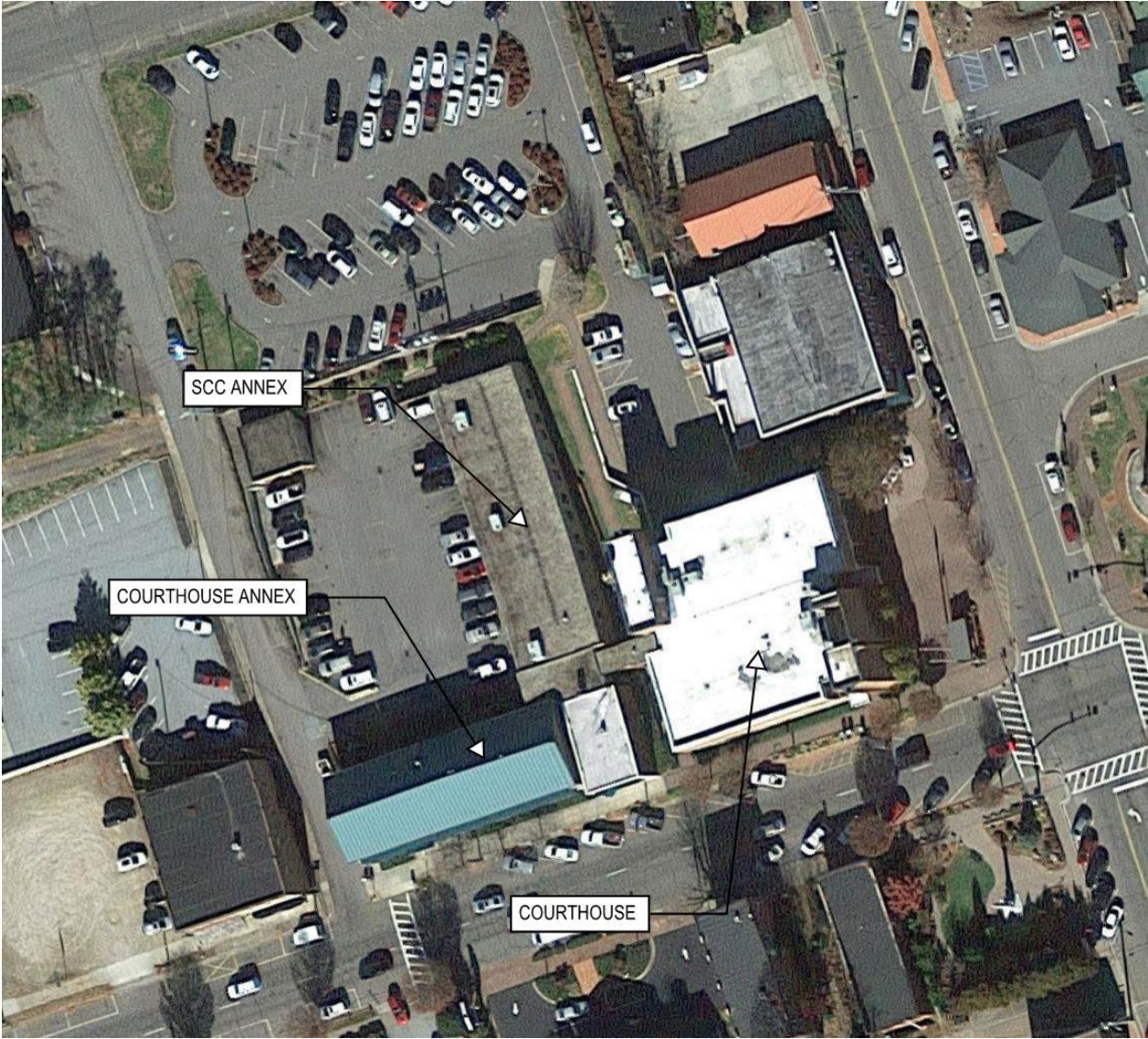
Fig. 2 – Overview of facility
