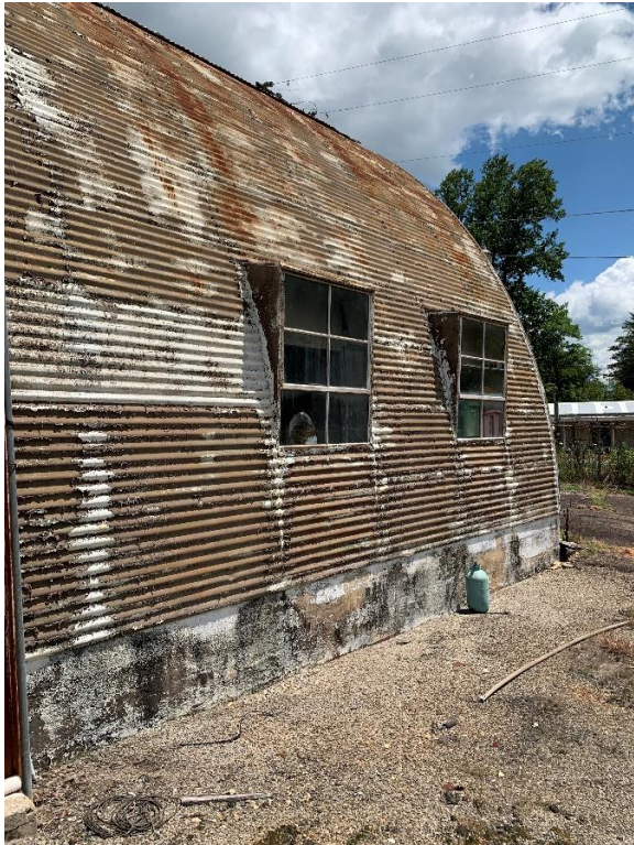
Fig. 2 – Overview of facility
