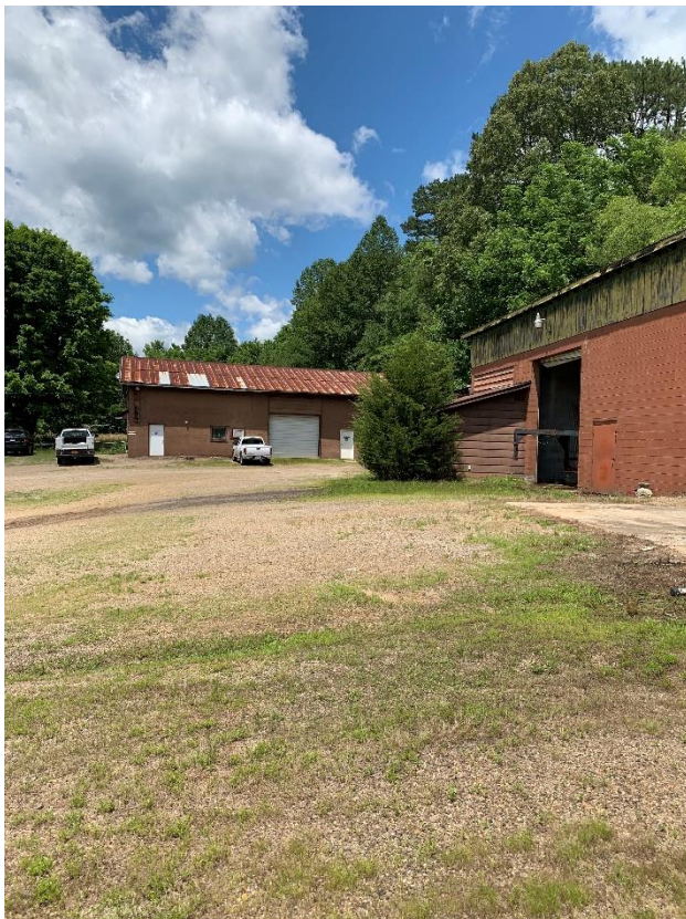
Fig. 1 – Overview of facility
