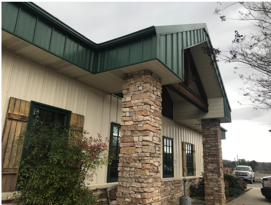
Fig. 1 – Overview of facility
